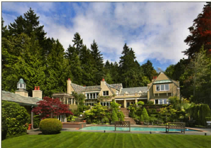
The new wing, on the right in this view of the back of the home, looks as though it has always been there. The conservatory, also new, is on the left.
