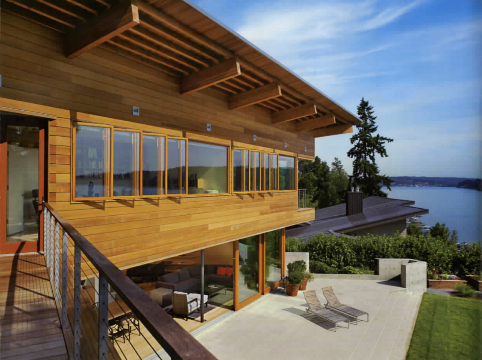
Upstairs are bedrooms, baths, a study and three decks. The deck at left provides a lookout over the terrace, as well as steps down to a hot tub and swimming pool. The chaises on the terrace are from Ikea.
