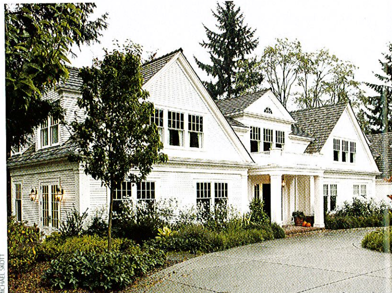
SCHULTZ MILLER BUILT THIS CUSTOM TRADITIONAL-STYLE HOME, DESIGNED BY STUART SILK ARCHITECTS, IN CLYDE HILL.
