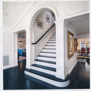
The new staircase (previously off-center, and cut off by an upstairs closet) takes center stage under a gracefully high new arch. "Moving the stair would have been too expensive, so it was widened to maintain the existing load paths while achieving symmetry in the space," says Anderson. "This stair is now the focal point of the home, with the new kitchen, family and dining rooms situated around it."
